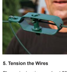
Place wire tensioners about 20 inches from the corner post, aligning them. Then, tension the top and bottom wires so they are taught. You should be able to clearly see your fence line at this point.
